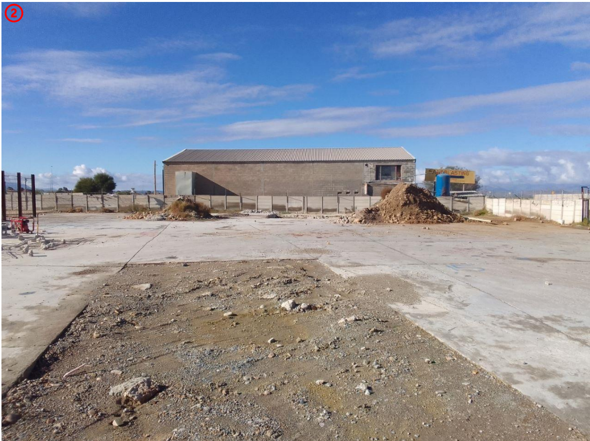
Photograph 2: Facing the south-eastern boundary of the site.
