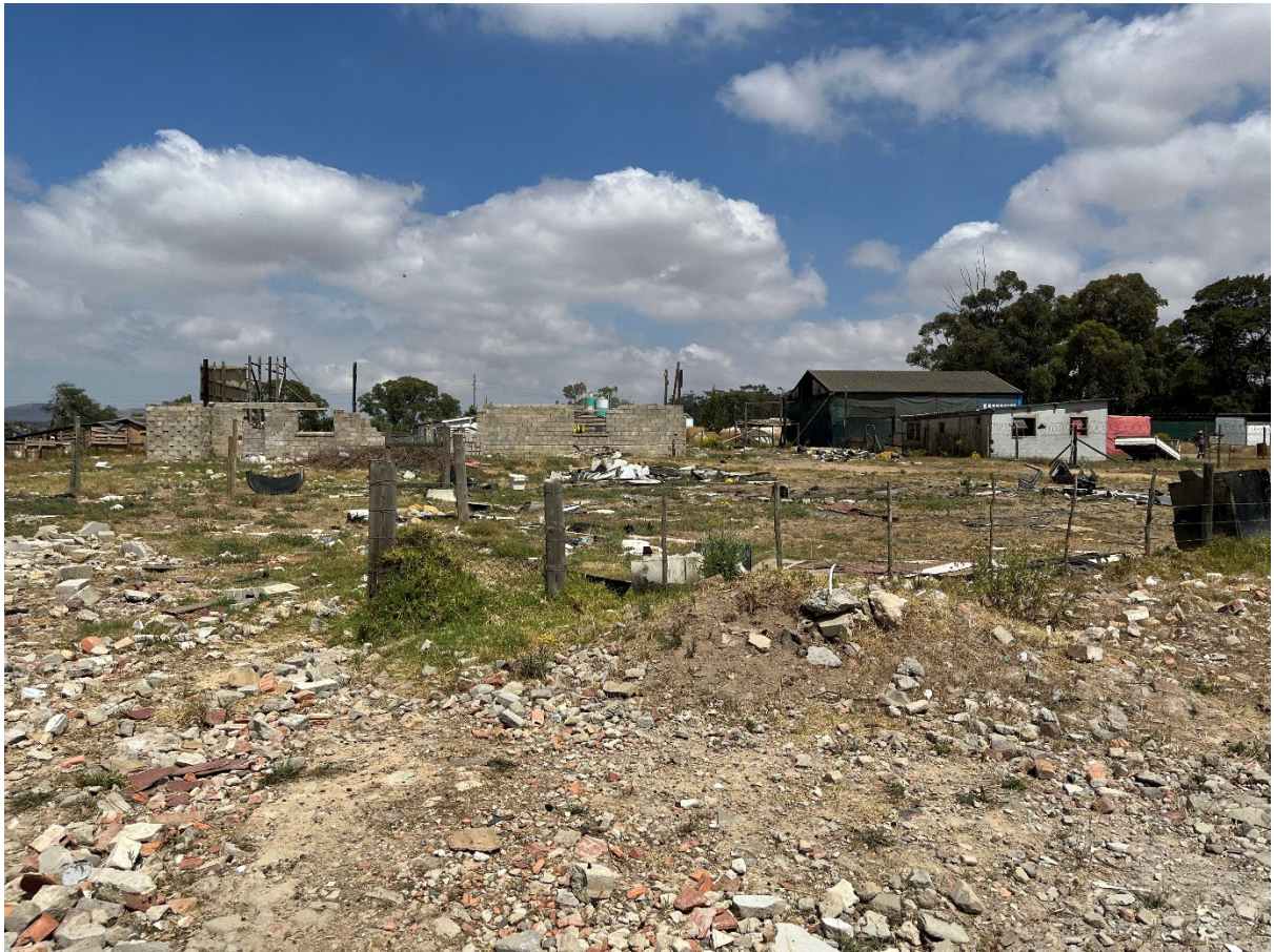
Photo 9: View across the site facing west, showing some of the existing structures on the site.
