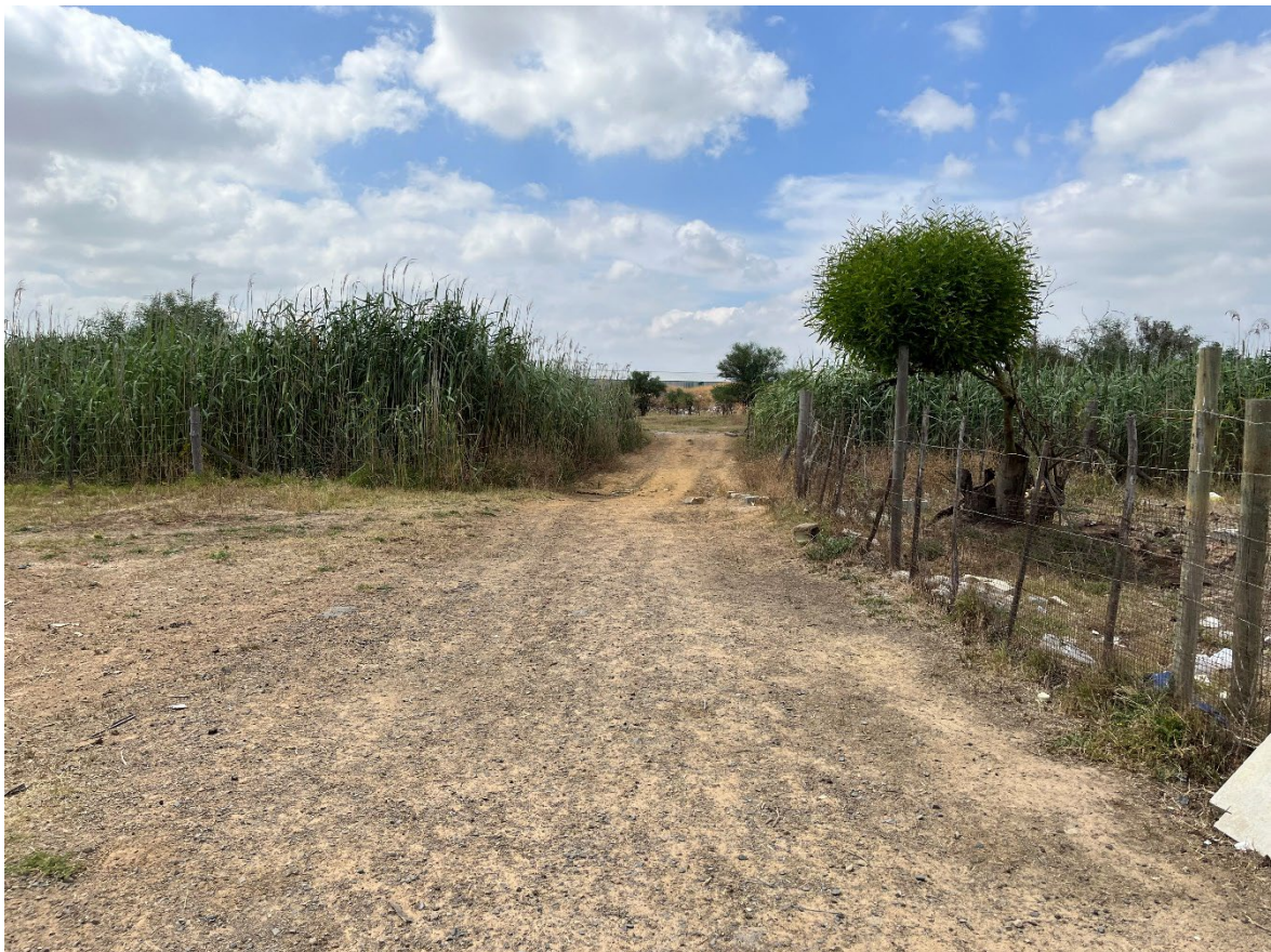
Photo 4: The existing low water crossing over the Mosselbank River tributary.
