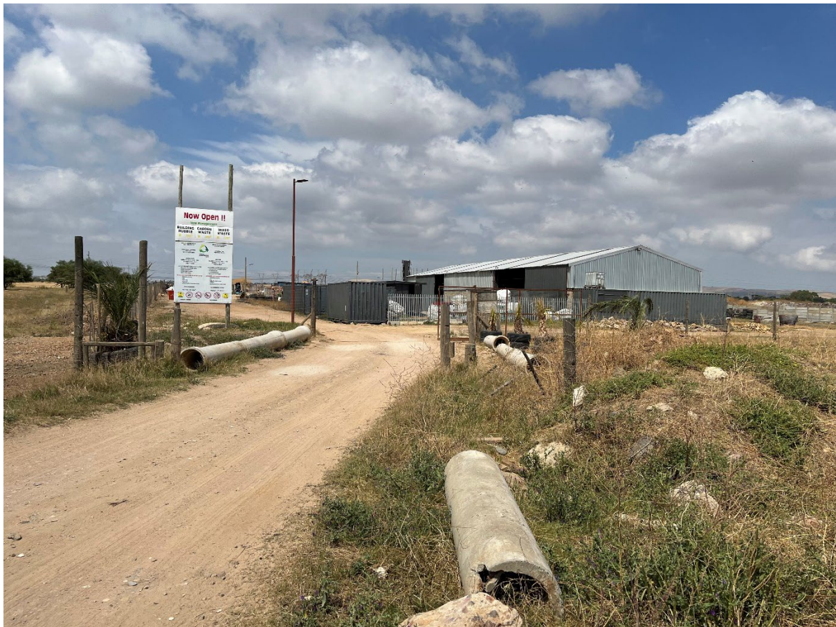
Photo 7: A recycling facility is located on the southern portion of the site.
