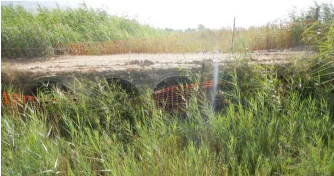
Figure 19. The pipe culverts under the road across the unnamed tributary in the middle of the property
