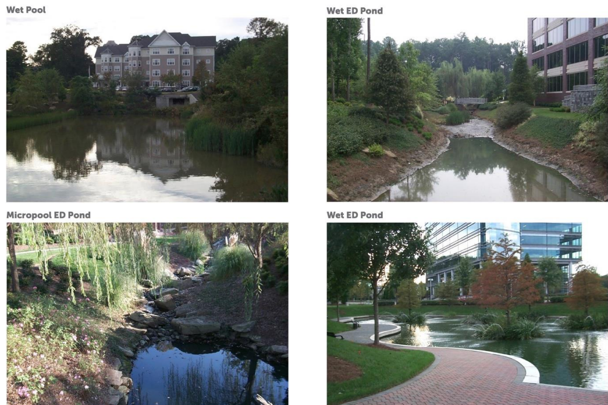
Figure 4: Photographs of Wet ponds (Ref. 2)
