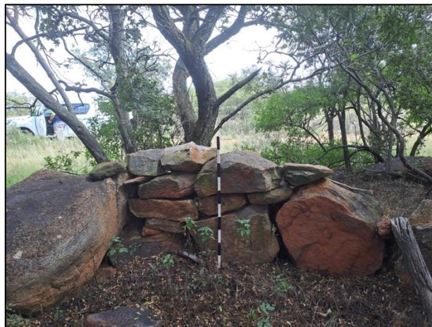
Figure 12 - View of the stone walling identified at CTV02.
