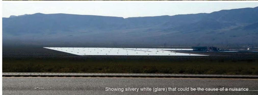
Apparent colour changes with differing sun angles and viewing geometry at a PV facility. (USDI 2013:78) Credit: Robert Sullivan, Agganis National Laboratory.
