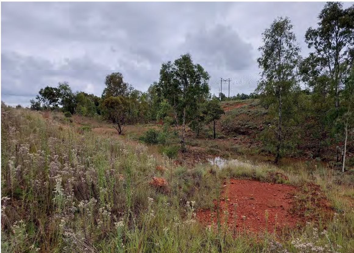
Figure 5-18: Excavations/diggings present along the eastern boundary of Portion 27 of Farm Doornfontein No. 118.
