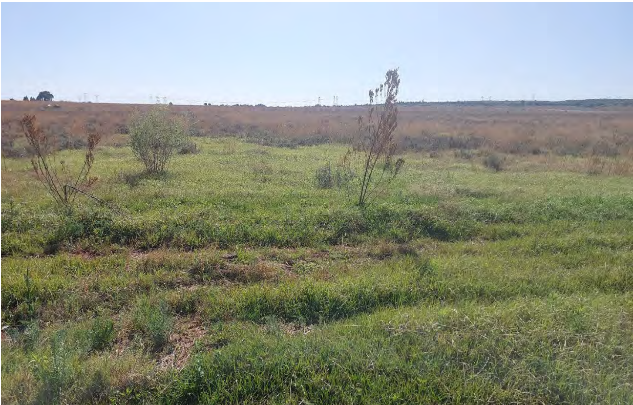
Figure 5-8: Upstream of the culvert located along the western border of Portion 5 of Farm Varkenlaagte No. 119.
