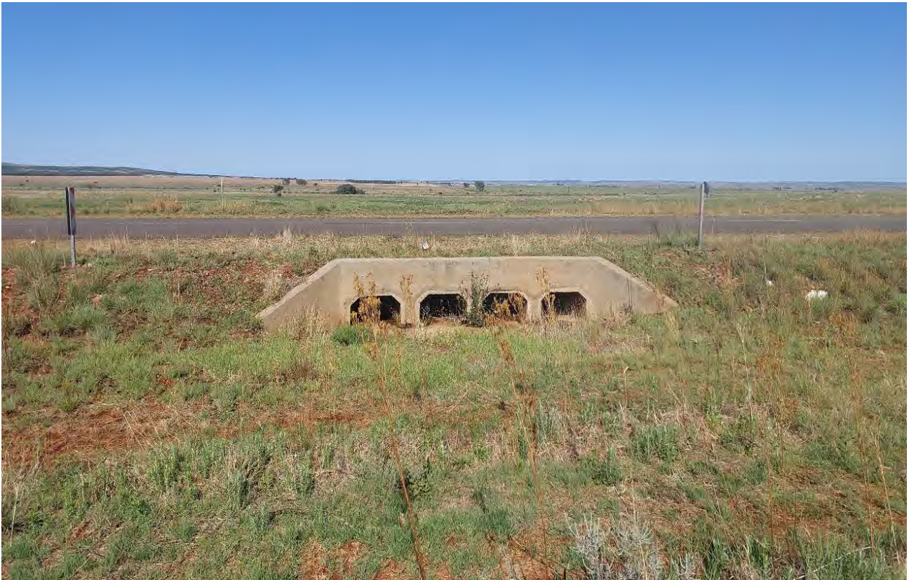
Figure 5-7: Culvert located along the western border of Portion 5 of Farm Varkenlaagte No. 119.
