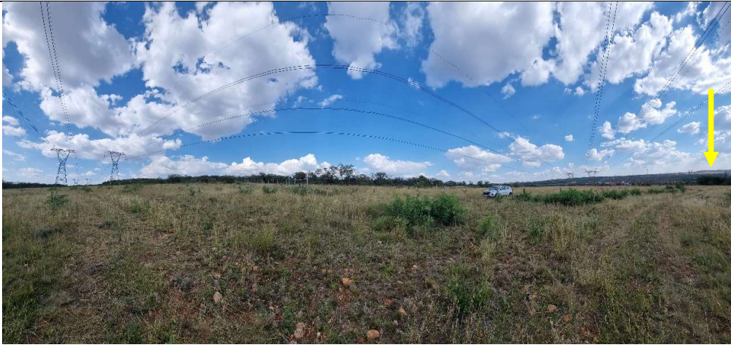
Photo 1: Panoramic image taken facing east, from the southern boundary of the site, relative to the Carmel substation (indicated by the yellow arrow).
