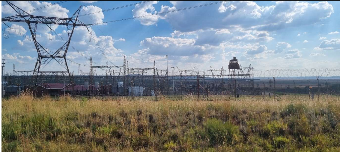
Photo 13: View of Eskom's Carmel Substation taken from the east looking west towards the substation and existing infrastructure.
