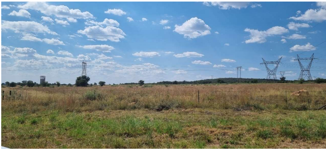
Photos 11 (top) & 12 (bottom): View of the existing pylons and overhead powerlines (OPL's) leading from the north/north-east, into the Carmel Substation.
