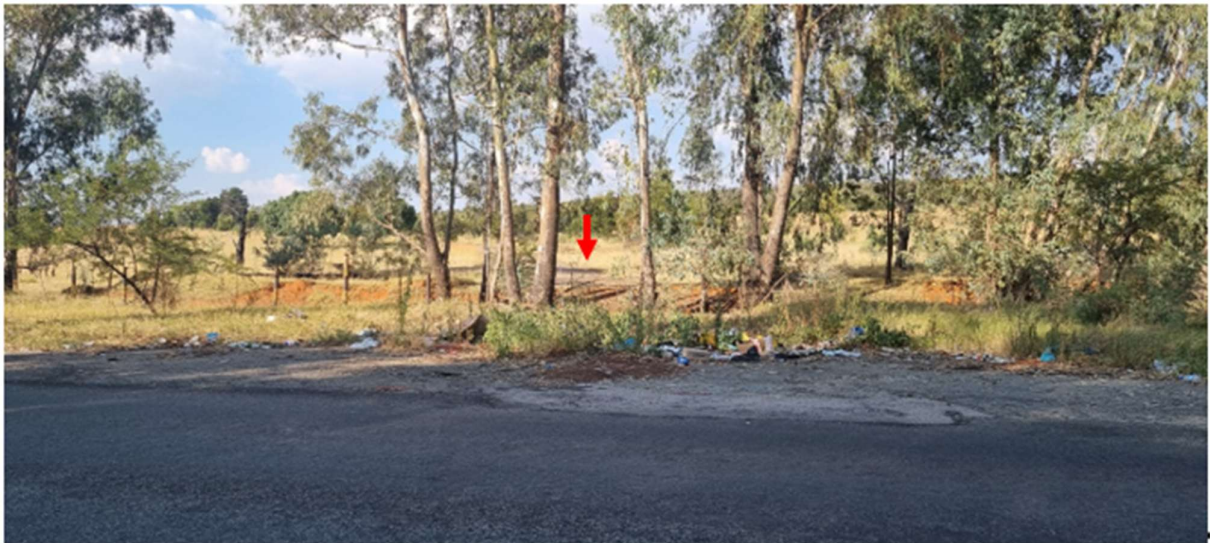
Figure 34: The original intersection of the public D92-1020 tar road running along the western boundary of the property (in the foreground of picture) with the main access tar road (indicated with red arrow) which crosses the development property from west to east. Actual entrance point not clearly visible from the D92-1020 due to excavation in the road reserve and vegetation growth.
