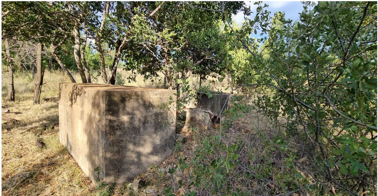
Figure 38: Concrete and brick structure on proposed development site (partially demolished).
