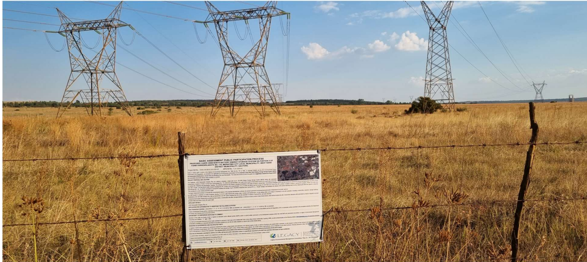
Figure 33: Eskom HV OPLs traversing the length of the development property from the north/north-east towards Carmel MTS in the south/south-west.
