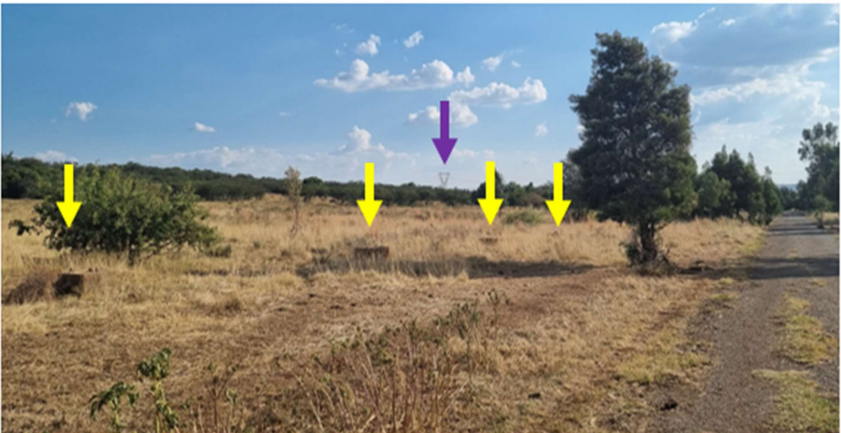
Figure 36: Evidence of concrete plinths (indicated with yellow arrows) which probably supported a conveyor belt or large pipeline leading to the mine dump to the immediate west of the proposed development site. Note the alien invasive trees (left of image) and plants (foreground), as well as the existing Eskom HV pylon (indicated with a purple arrow) which runs through the property.
